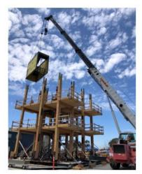
Left: Installation of Level 2 columns; Middle: Level 2 complete; Right: Installation of story 3 modular stair system unit with fire-rated wall panels.
